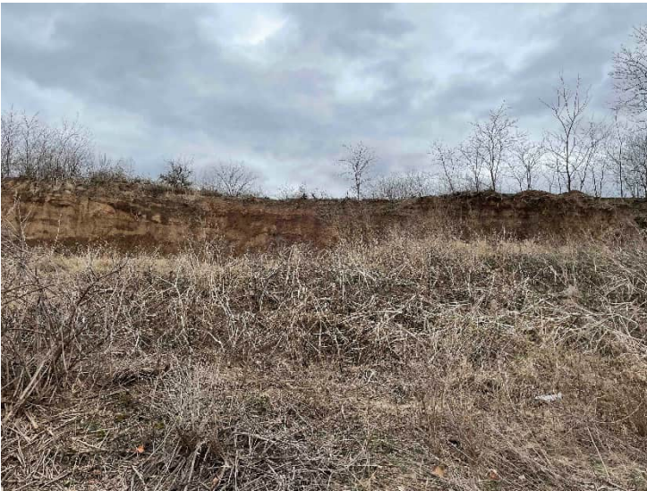
Photograph 9: Erosional slope found within the Brownleigh site
