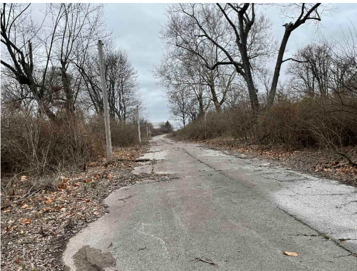
Photograph 6: General view of a road that intersects the Brownleigh site
